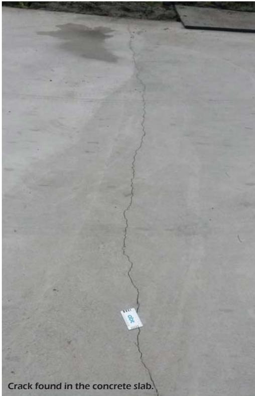
Crack found in the concrete slab.
