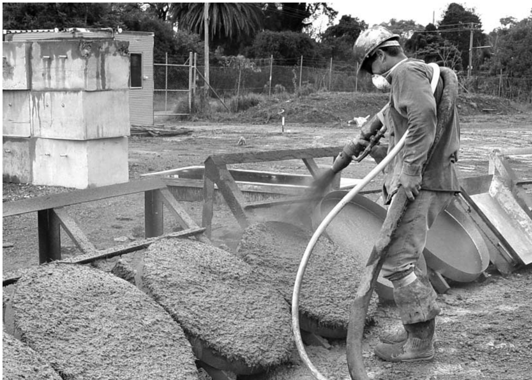
FIG. X1.5 Manual Spraying of Panels
