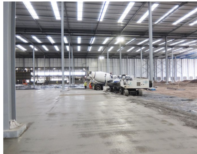
Slab construction
