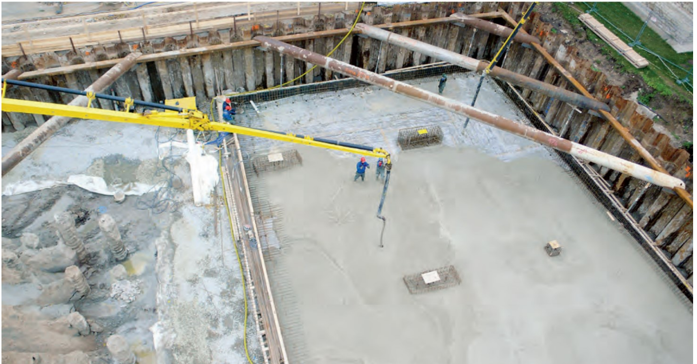
Piled-supported slab
