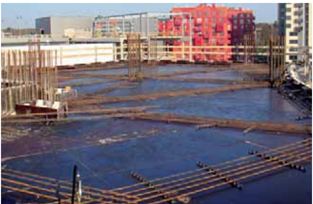
Figure 9: LKS office building with TAB-Slab pouring in progress; APC reinforcement is also visible.
