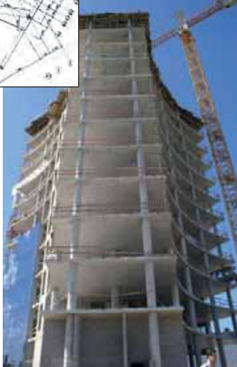
Figure 12 right: Rocca Tower – TAB-Slabs and concrete frame partially completed.
